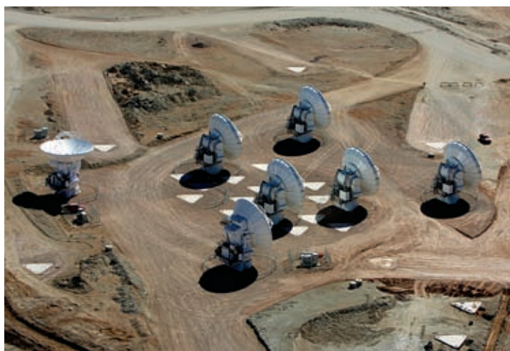
The Atacama Large Millimeter/submillimeter Array will consist of 64 movable 12-meter (40-foot) antenna dishes that can be arranged in patterns ranging from 150 meters (500 feet) to 16 kilometers (10 miles) wide. The specialized computer that combines the information received by the antennas will perform 16 quadrillion (16 million-billion) operations per second. Credit: NRAO/AUI and NRAO/AUI/NSF, Carlos Padilla, General Dynamics C4 Systems
