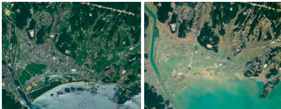
Before-and-after imagery from the GeoEye-1 satellite shows the damage at Rikuzentakata, on the Northeast coast of Japan, following the earthquake and tsunami in March 2011. According to police, every building less than three stories high was completely flooded. Credit: Images ©GeoEye Inc. Distributed by e-GEOS.
