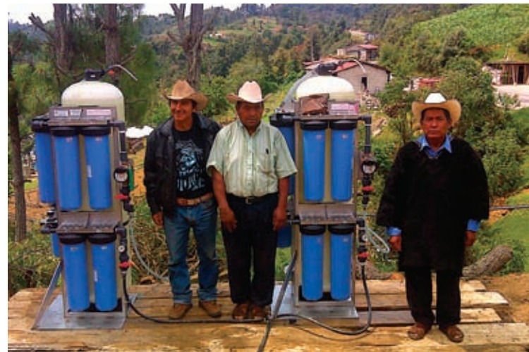
Community leaders in Cruz Quemada, Mexico, pose with a new water purification system designed by Water Security Corporation for use in remote locations. Hundreds of similar systems have been installed in rural villages around Mexico, reliably delivering safe, purified water from local sources. Water Security Corporation's proprietary technology is based on iodinated resins that have been used by NASA for nearly 30 years on the Space Shuttle and International Space Station. Credit: Water Security Corporation
