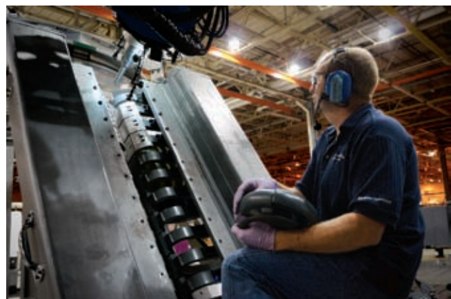
Construction begins with the first weld on the Orion Multi-Purpose Crew Vehicle (MPCV) at the Michoud Assembly Facility in September 2011. This is the first Orion capsule that will undergo a test flight in space. Credit: NASA
